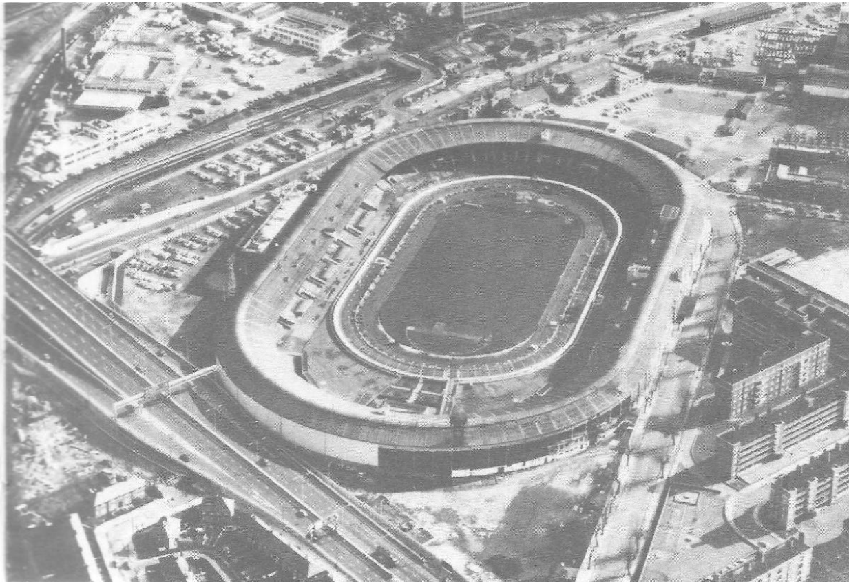
Aerial view of White City Copyright – GRA
